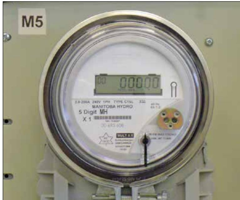
Pulse type load meter. This special meter monitored power consumption in the crates every 15 minutes, for an accurate picture of electrical demand and usage.
