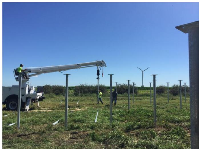
Figure 1. Installing Solar Array Earth Anchors
